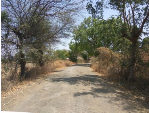
Fig.5 Road Condition in village
