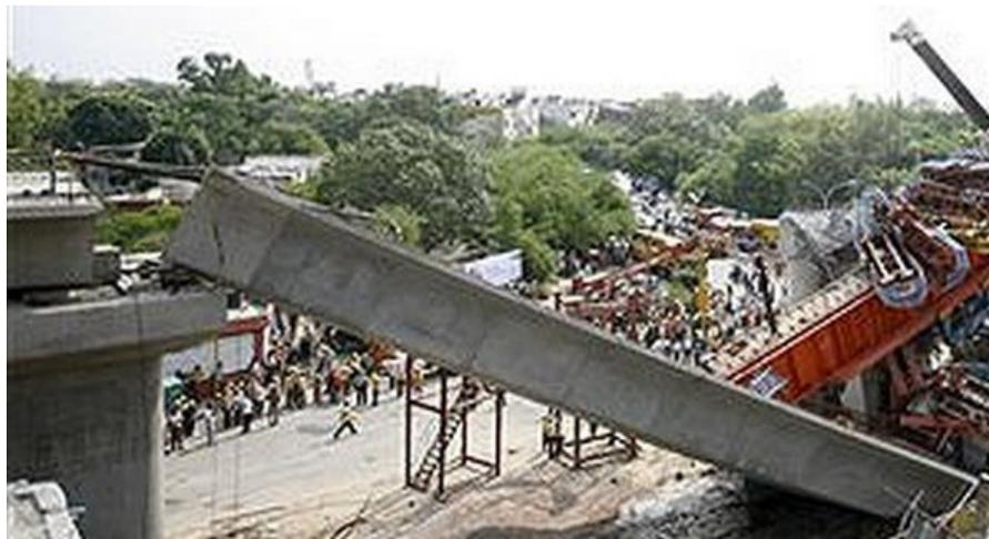
Fig.2 Elevated section of the tracks under construction came crashing down in Delhi Metro
