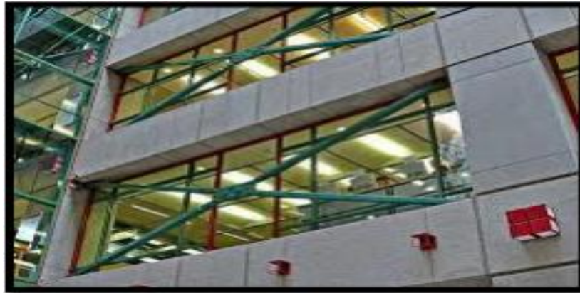
Fig.4 Friction Damper
