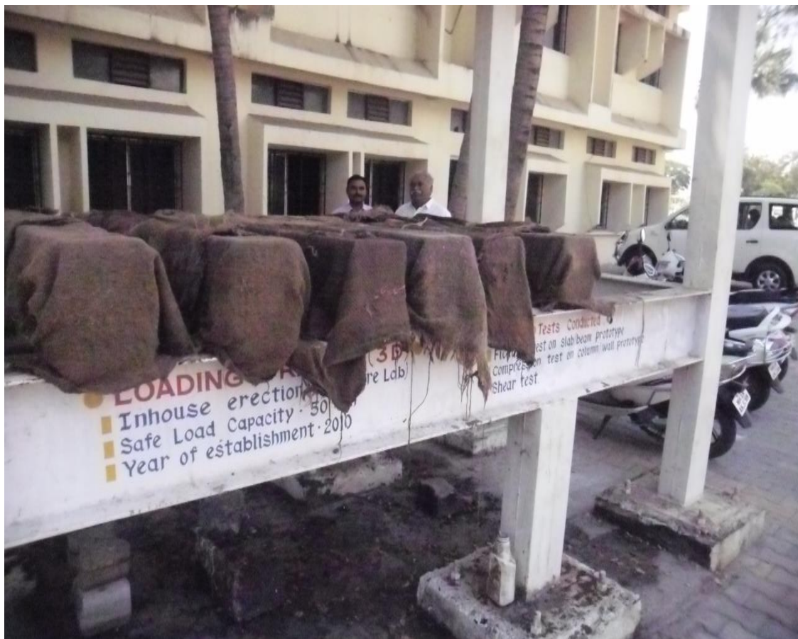
Fig 5. Curing of Casted RCC Beams
