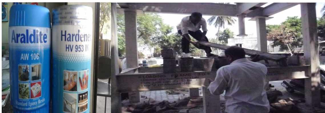
Fig.7 Bonding of beam soffit with SIFCON Laminates.
